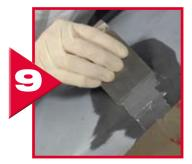
Spread and smooth 3M™ Flexible Parts Repair Material 05901 into the crack and allow to dry for 20 minutes.
