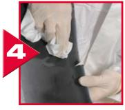
Clean the area using 3M<sup>™</sup> VHB<sup>™</sup> Surface Cleaner or 3M<sup>™</sup> General Purpose Adhesive Cleaner 08984 applied with a 3M<sup>™</sup> Professional Panel Wipe 34567.
